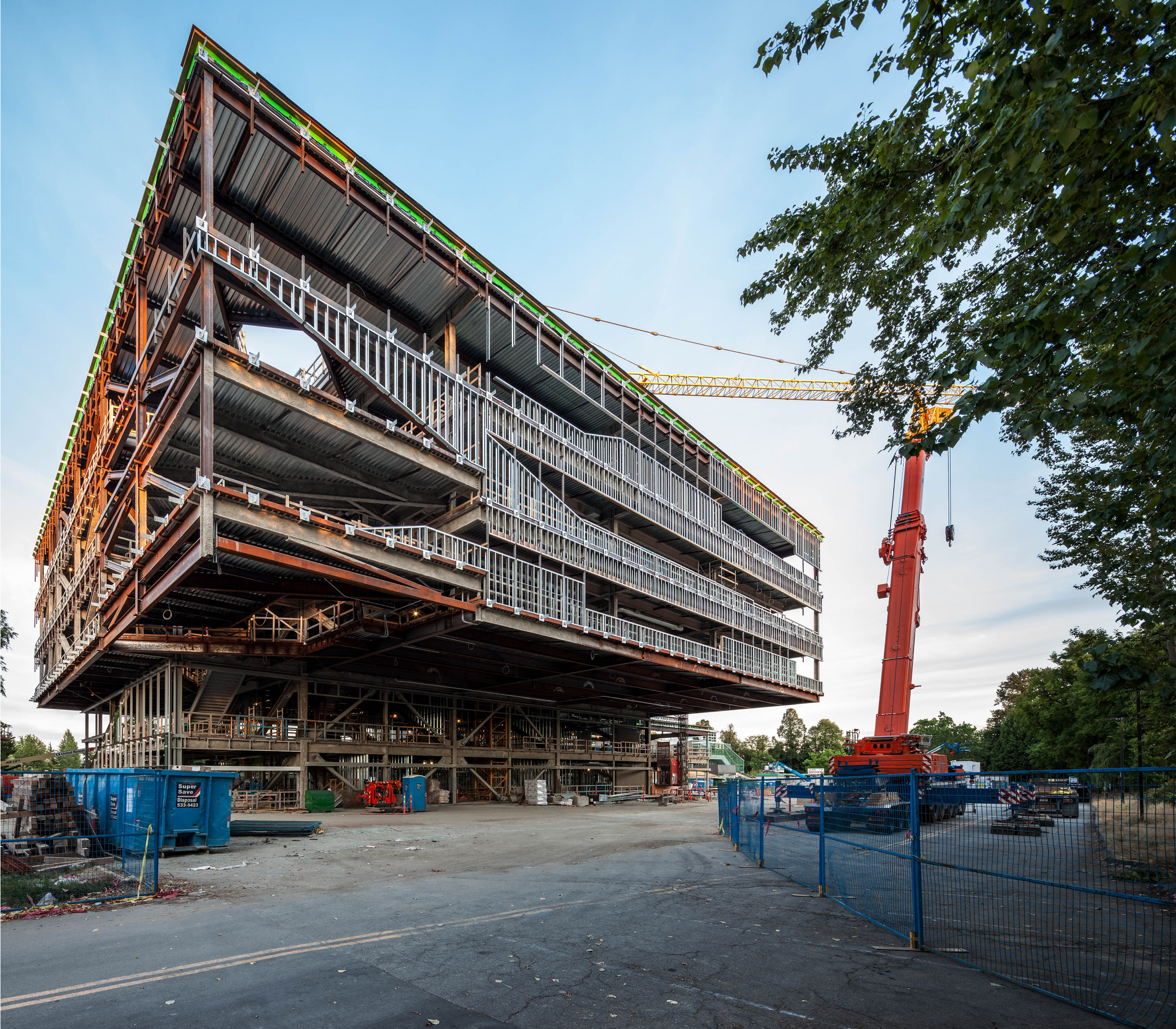
Steel Cantilever System Supports Floors Above
