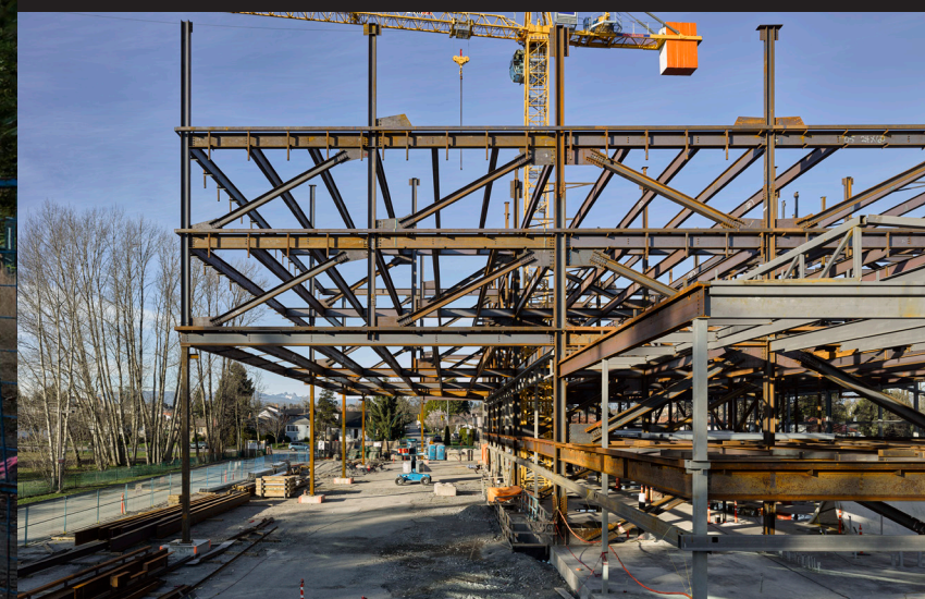
Steel Cantilever System Supports Floors Above
