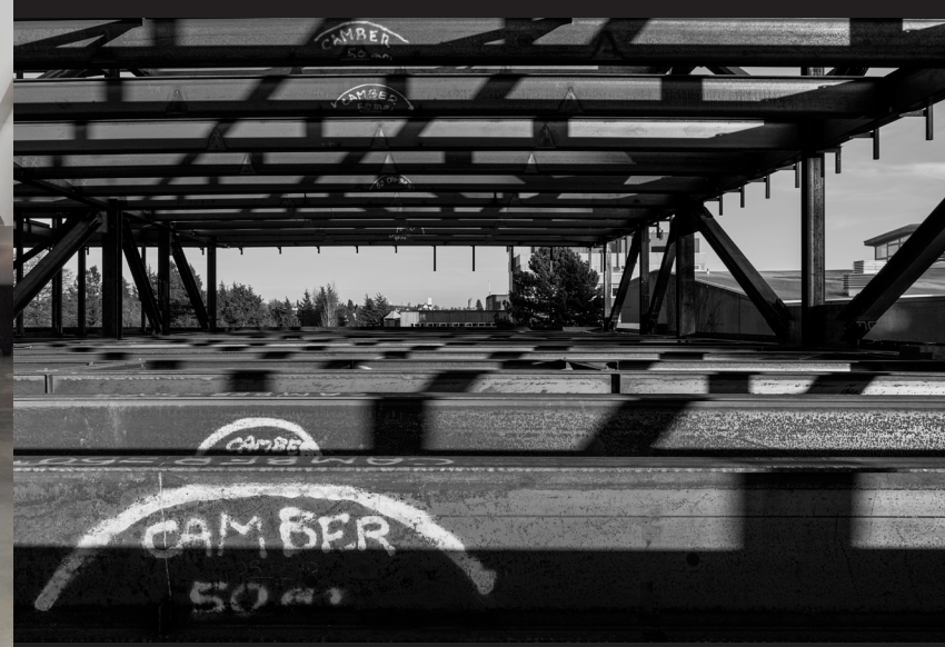
Steel Trusses - Building used 1,600 Tons of Structural Steel
