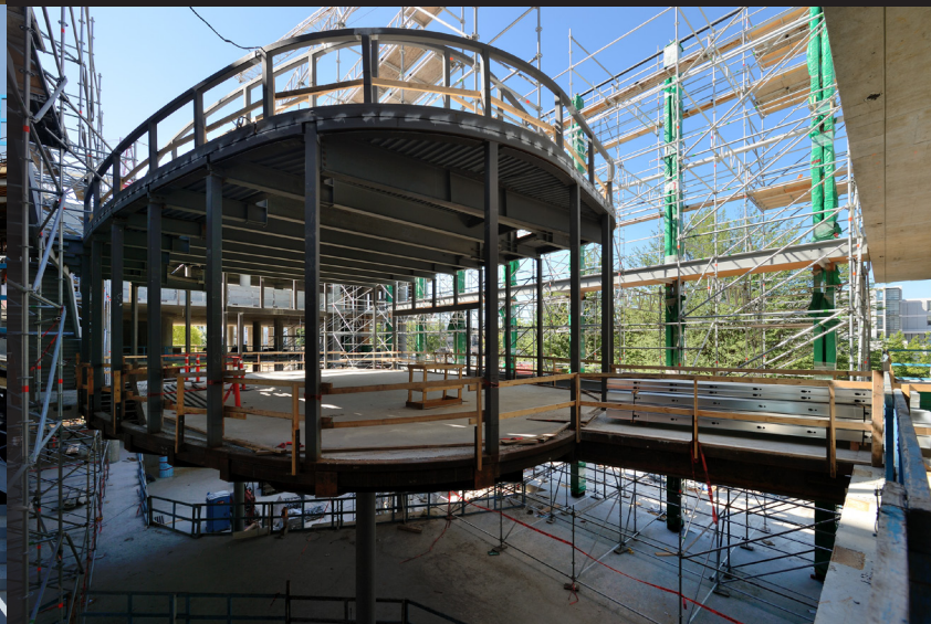
Nest: Core Floor Structural Frame on Slender Steel Supports
